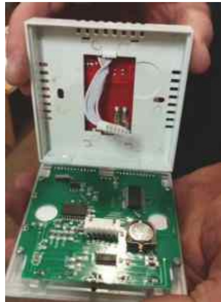
5. The screen can be put to one side for re-connection later. The body of the stat can now be wired and fixed back into the wall box.
